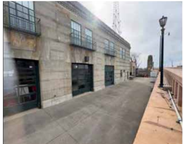
Beautiful windows after installation.
