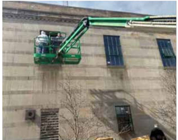
Work crew installing windows on the second floor.
