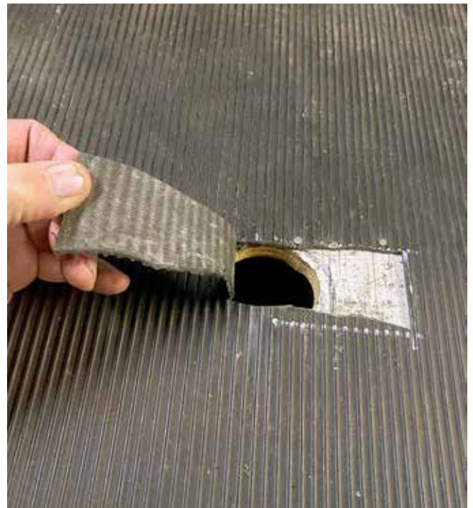
We now have an access point so that the master cylinder cap can be removed, master cylinder fluid level checked and brake fluid added as necessary. Photos by Tommy Herman.
