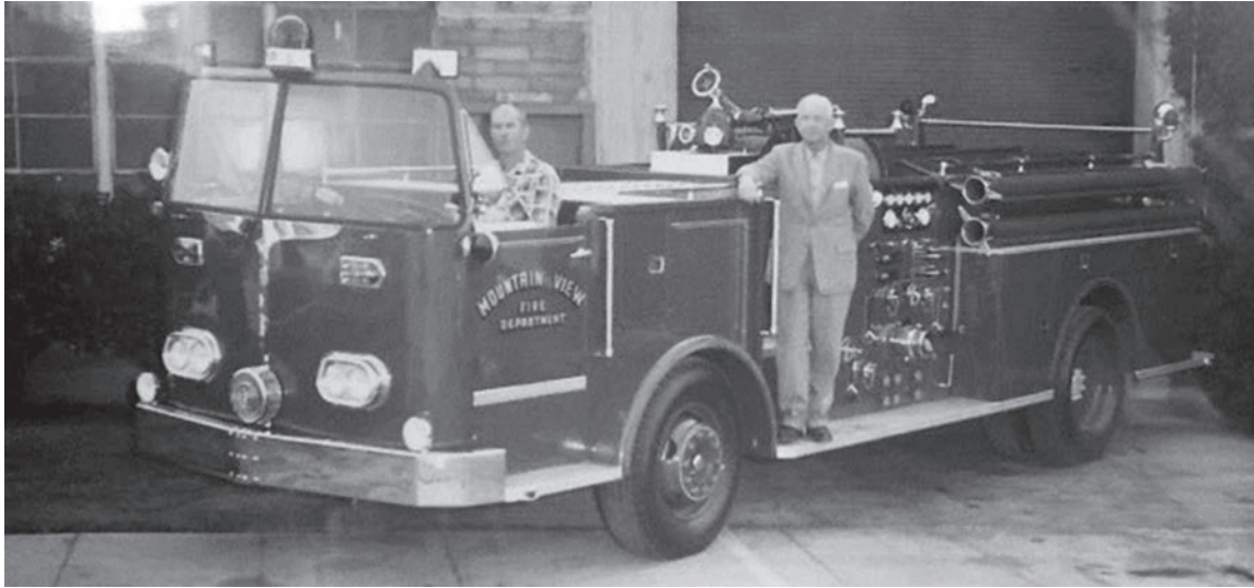
George Chappell, designer of the Van Pelt Custom 300, behind the wheel, and P.E. Van Pelt on running board of the first Van Pelt Custom 300 fire engine, serial #1412, completed for Mountain View, CA in 1960. The heavily modified chassis started out as a Diamond T in 1958. All subsequent Custom 300s used Van Pelt's own custom chassis, built in-house. Lynn Chappell collection.
