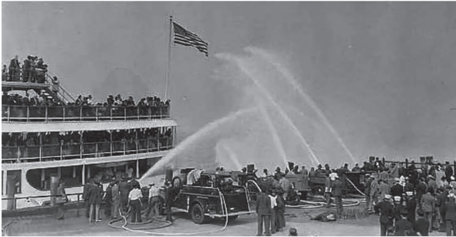
FDNY conducted a test of 500-gpm trailer pumps from eight different manufacturers in August of 1941. Photo from the John Calderone Collection.
