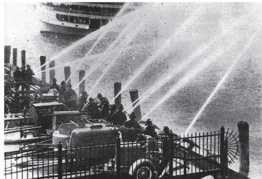
FDNY conducted a test of 500-gpm trailer pumps from eight different manufacturers in August of 1941. Photo from the Alex Black Collection.
