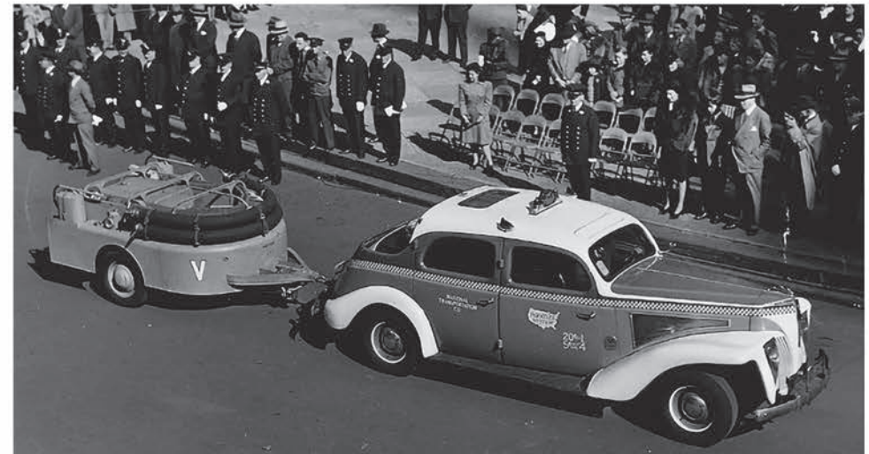
In the photo above, New York City appears to have made arrangements for the trailer units to be towed to the fire scene by taxis as shown in this demonstration. Photo from the John Calderone Collection.
