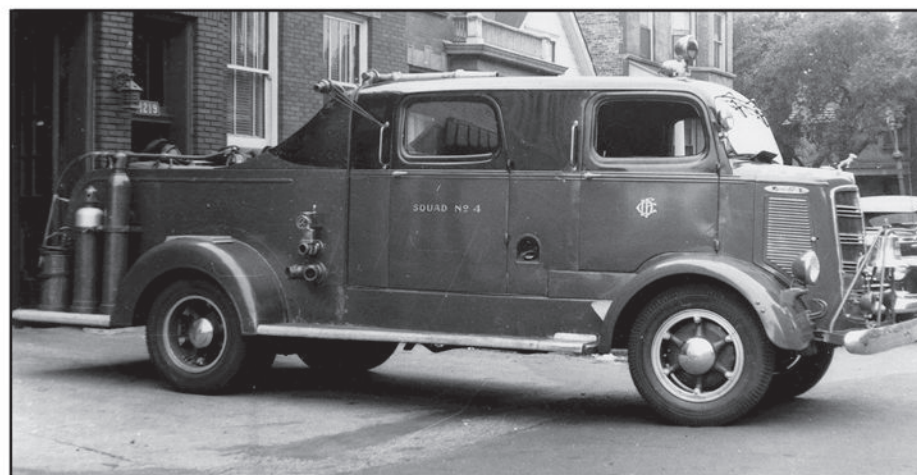
Chicago purchased 12 of these 1941 Type 45U "squad cars" that were built on a cab-over-engine version of the E Model with four-door cabs. Bob Freeman photo.
