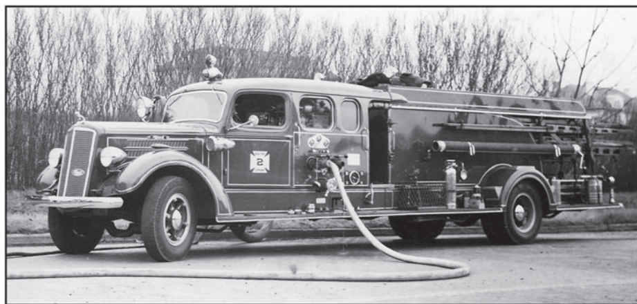
Mack's skilled craftsman in Long Island City built many interesting custom apparatus. Among these is this 1941 Type 505 quadruple combination with a "special 6-7 man canopy cab with side openings." It served in Deal, New Jersey.
