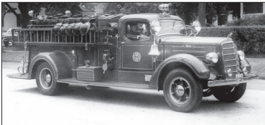
Mack's Pre-War production in Long Island City was brief, but included a wide variety of apparatus. This 1941 Type 45 triple combination pumper with a coupe cab and a 500-gpm pump, served in Greenport, which is at the eastern end of Long Island, about 95 miles from the Long Island City facility.
