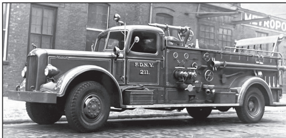
Despite wartime restrictions on the production of civilian fire apparatus, the FDNY received ten Type 21-LS pumpers in May 1944. These had coupe cabs, 1,000-gpm Hale pumps and 2000-gpm Morse deck pipes.
